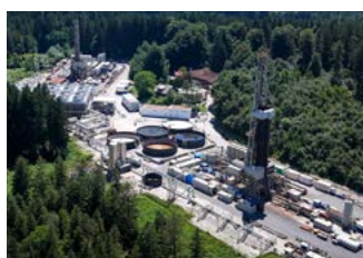
Eavor Technologies ~$138M | CLEANTECH Alberta
